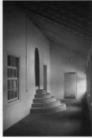
(b) Strip, staff-went coast, built about the same time ('foundation', A.J.A. Schrevers 1983). Rear gallery with 'Serlio' stairs in yellow brick, leading to the steep wooden stairs to the bedrooms under the roof, ventilated by the nearby breezes (TG 1981).
