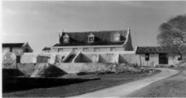
(b) Strip, staff-went coast, built about the same time ('foundation', A.J.A. Schrevers 1983). Rear gallery with 'Serlio' stairs in yellow brick, leading to the steep wooden stairs to the bedrooms under the roof, ventilated by the nearby breezes (TG 1981).
